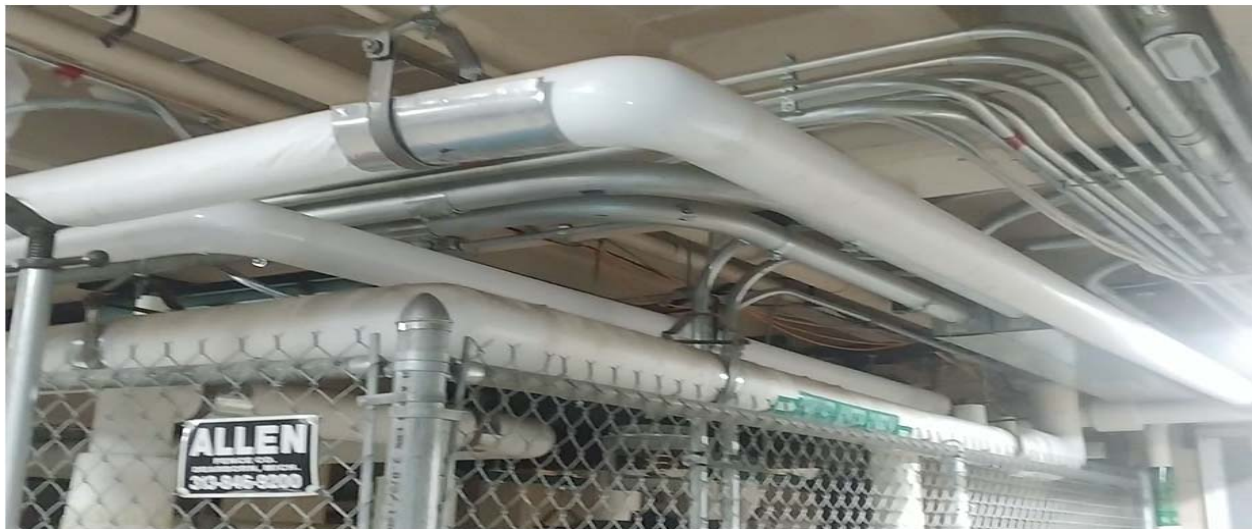
New piping and old piping future connection.
