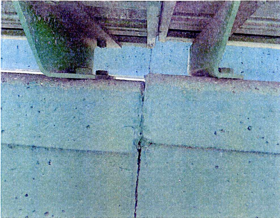
5. The north bleacher has been raised due to formation of pack rust at the bearing plates.
