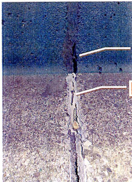
4. Failed sealants between the precast concrete panels.
