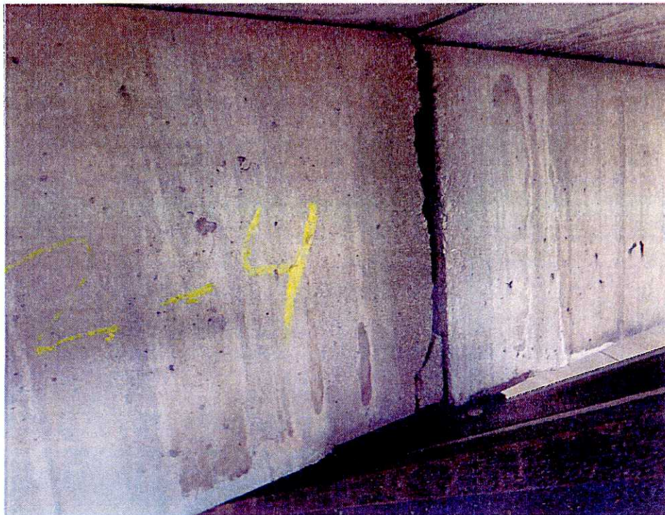
2. Column Line 2, Row 4: The north bleacher contains a minor concrete spall.
