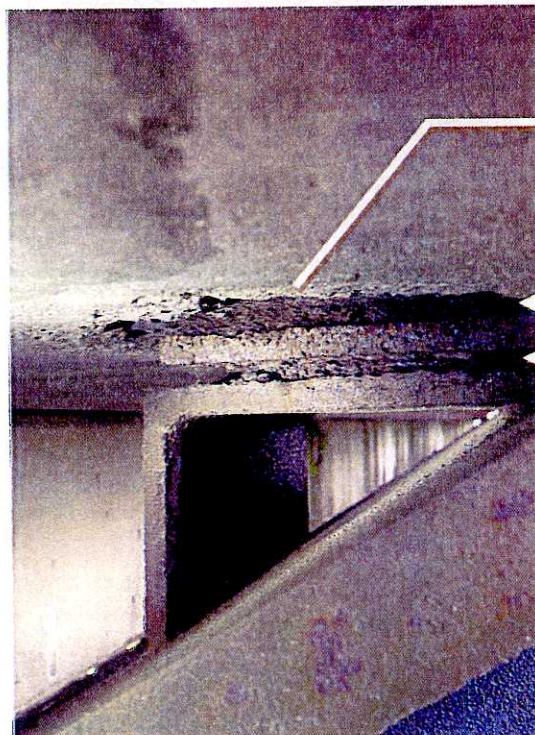
8. Pack rust between the two plates (red) and pack rust between the plate and concrete (blue)
