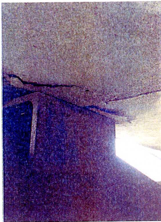
7. Notice the spalling concrete around the bearing plate. Typ.
