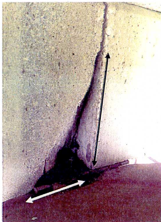
10. Column 3, Row 34: 6" (white) by 8" (black) corner spall.
