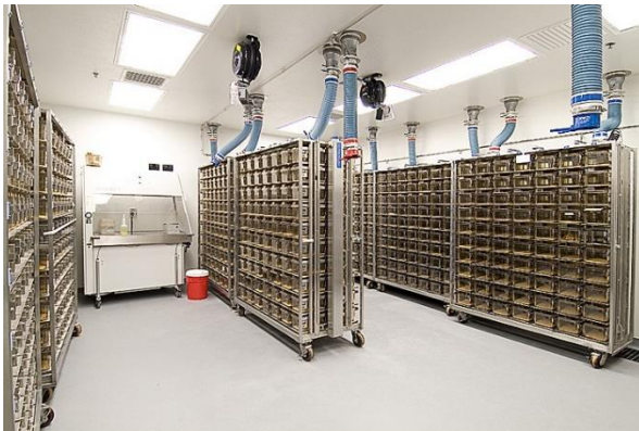
Typical Holding Room for Mice with Single & Double Sided Ventilated Cage Racks
