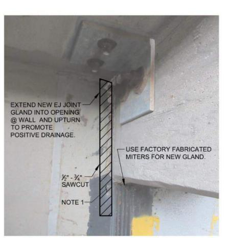
EXISTING SLAB IS POURED TIGHT TO COLUMN. REMOVE CONCRETE TO CREATE NEW BLOCKOUT TO EXTEND EJ SYSTEM AROUND COLUMN TO WALL. SEE DETAIL 10.3.1 FOR EJ DETAIL @ COLUMN.
