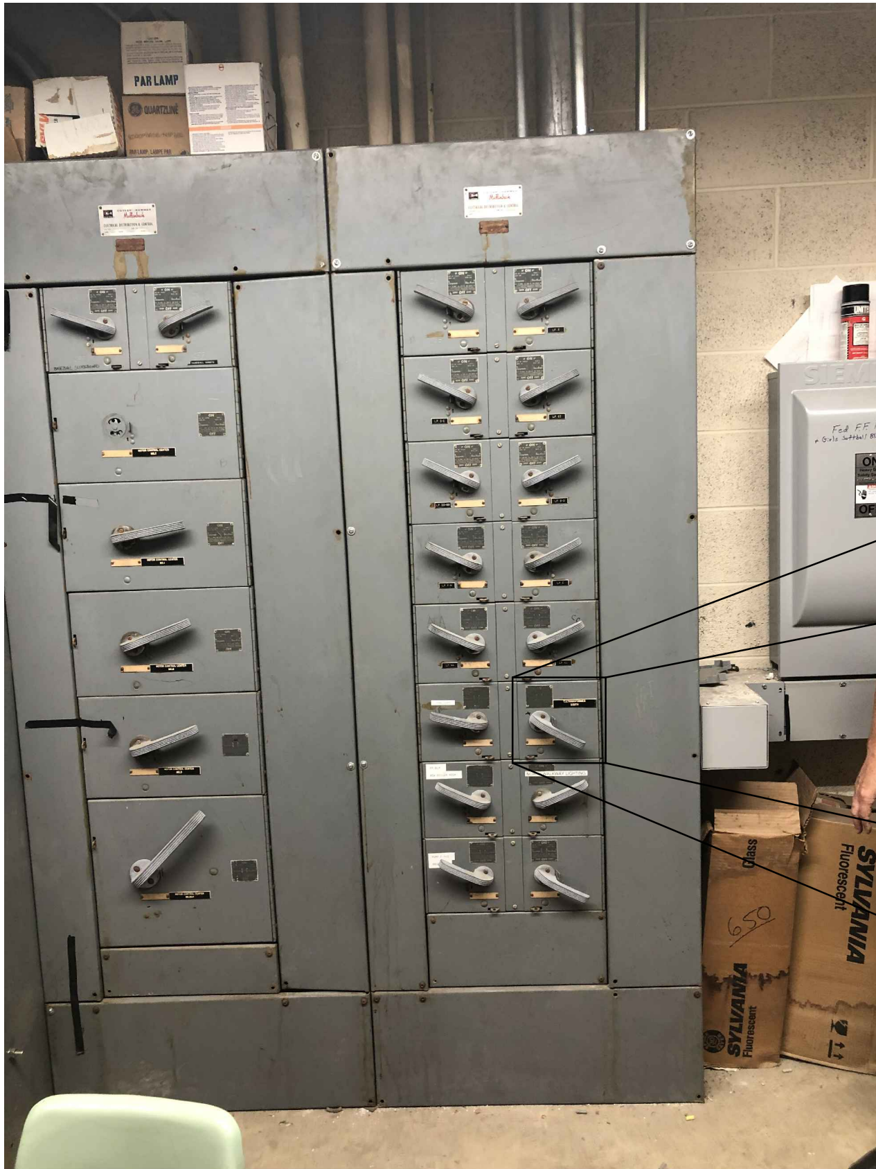
(E)MAIN SWITCHBOARD 480Y/277V 3ø, 4W, 1200A
