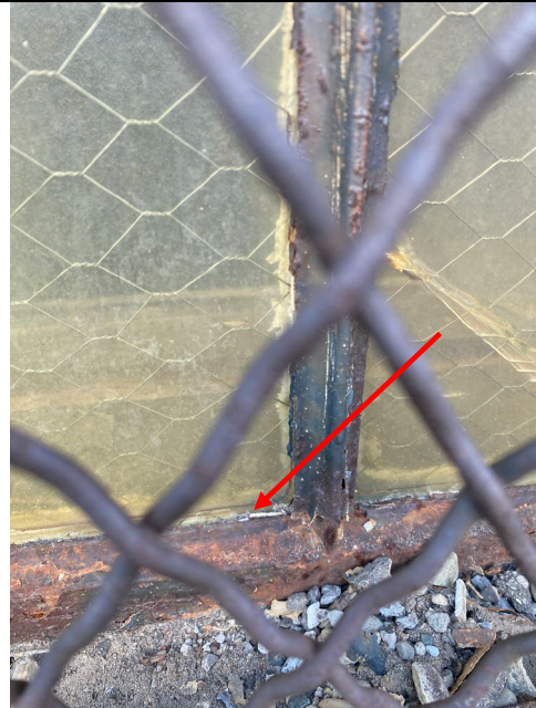
HM#36 Asbestos-Containing Window Glaze (Grey)
