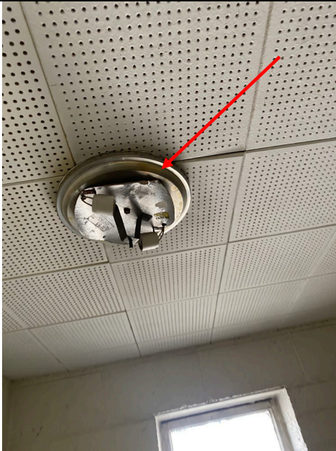
HM#24 Asbestos-Containing Light Heat Shield (Grey)
