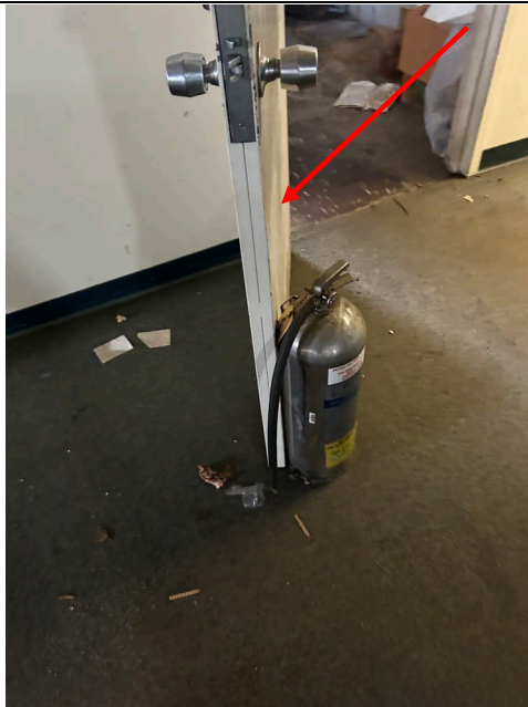
Assumed Asbestos-Containing Fire Door
