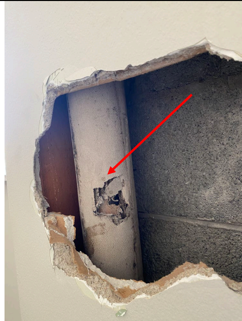
HM # 11 Asbestos-Containing 4" Straight Pipe Insulation (Grey)
