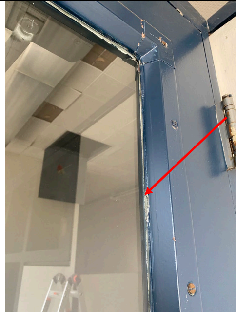
HM#5 Asbestos-Containing Interior Door Window Glaze (Grey)
