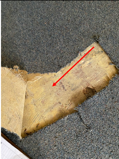
HM#8 Asbestos-Containing 9"x9" Floor Tile (Tan) w/ Adhesive (Black)& Adhesive (Yellow)
