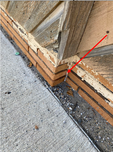
HM#24 Asbestos-Containing Light Heat Shield (Grey)
