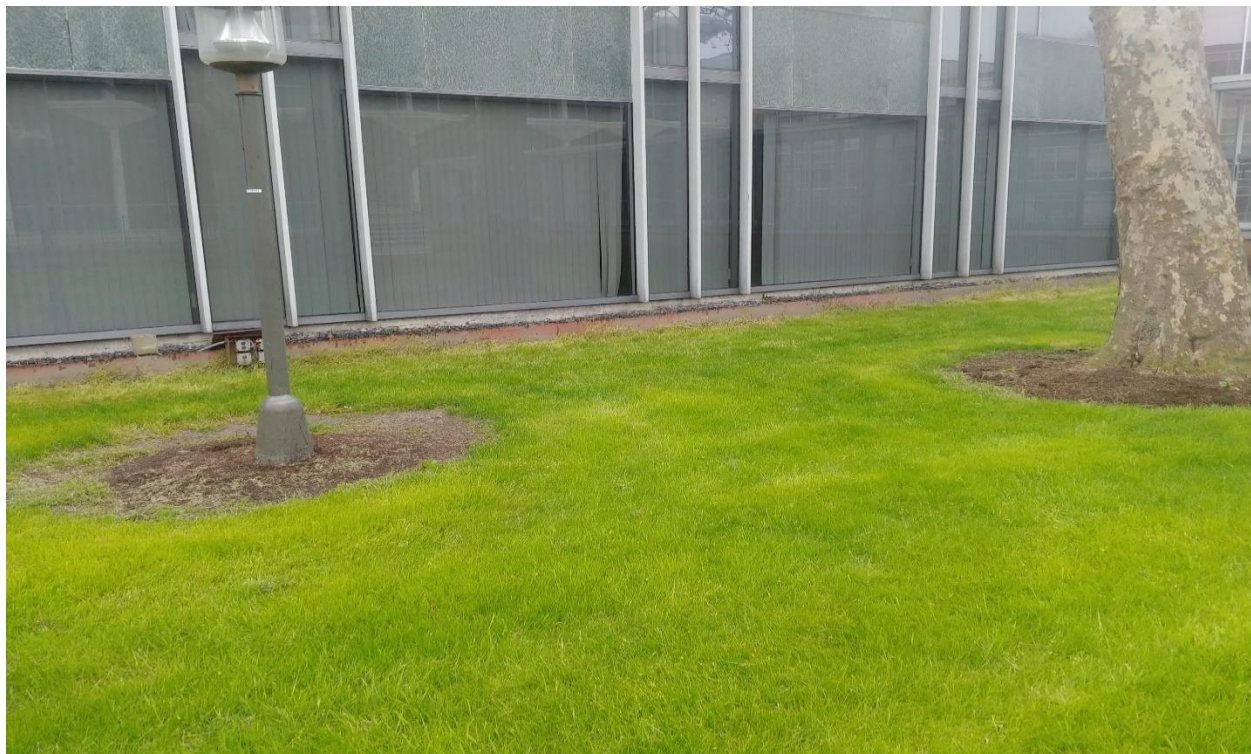
New chiller location
