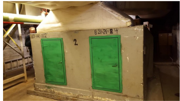
013A AHU-002 Filter Section
