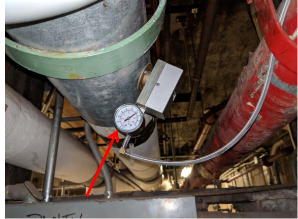
012B - TC-2.7 Chilled Water Temperature Sensor
