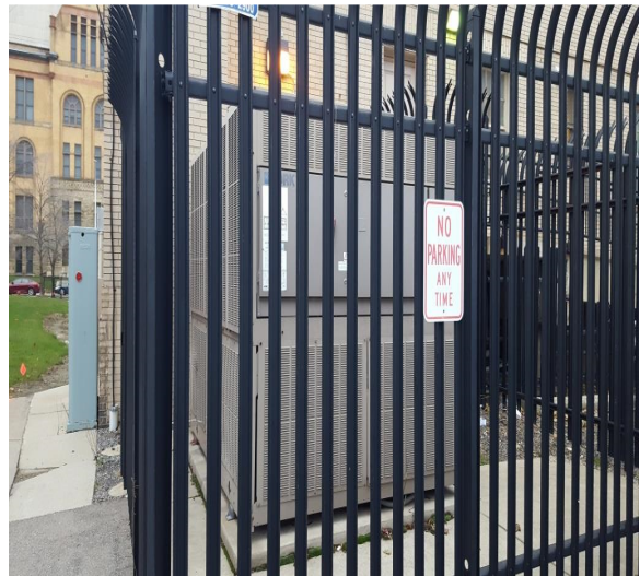
023 Chiller Air Cooled Condenser
