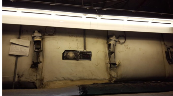
014 AHU-002 Damper Controls
