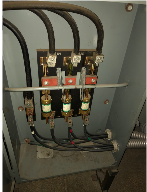
E16B Dimming Rack Disconnects
