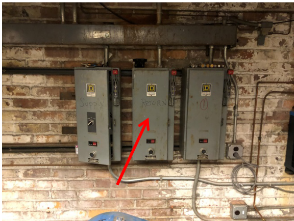
012C - HVAC-2.14 Return Fan Disconnect
