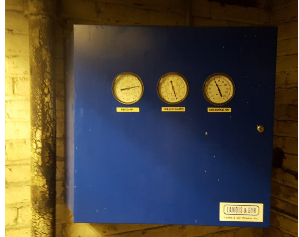
011 Pneumatic Control Panel
