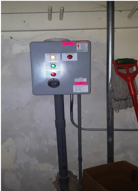
022 Sump Pump 3 Controller
