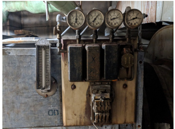
028C - TC-1.3 AHU-1 Heating Coil Control
