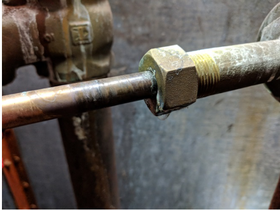
028F - HVAC-1.9 AHU-1 Leaking HC Isolation Valve
