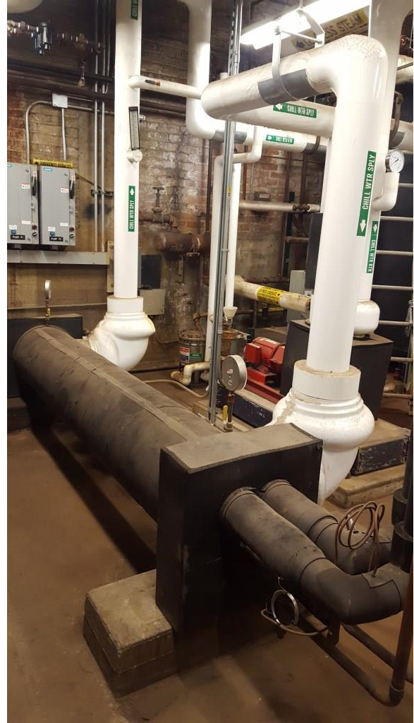
006 Chiller Heat Exchanger
