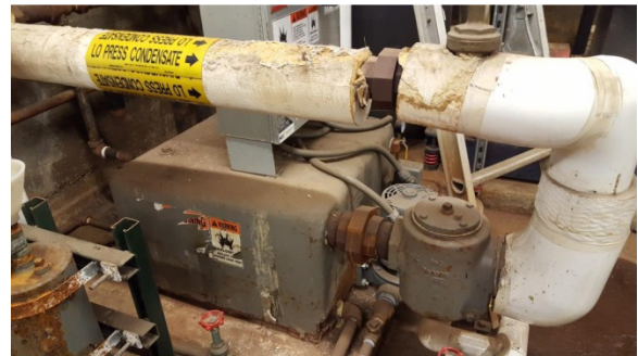
008 Steam Condensate Receiver
