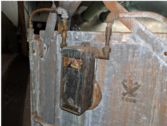
028B - TC-1.2 AHU-1 Bypass Damper Control
