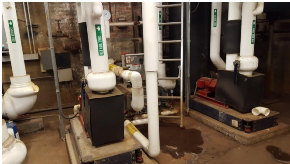
007 Chilled Water Pumps P-1 and 2
