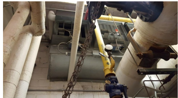
004 Combustion Air Unit
