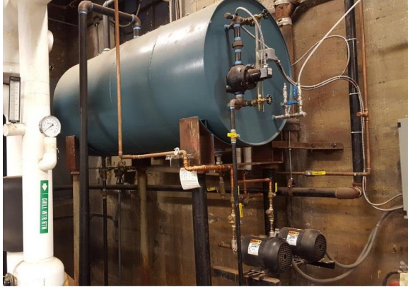
009 Condensate Transfer Tank
