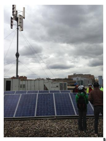
The Engineering Technology Building at Wayne State University features a vertical wind turbine and solar array. The energy generated by the alternative energy system powers one of the building's computer labs.
