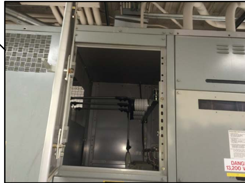
1b DTE ENERGY METERING SECTION SCALE: NONE
