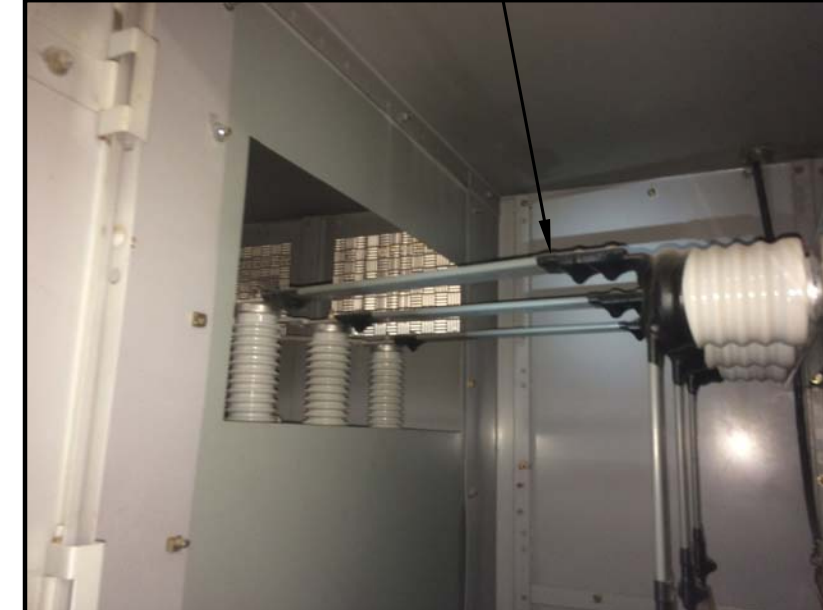
1c DTE METERING SECTION TEMPORARY CABLES TERMINATION LOCATION SCALE: NONE
