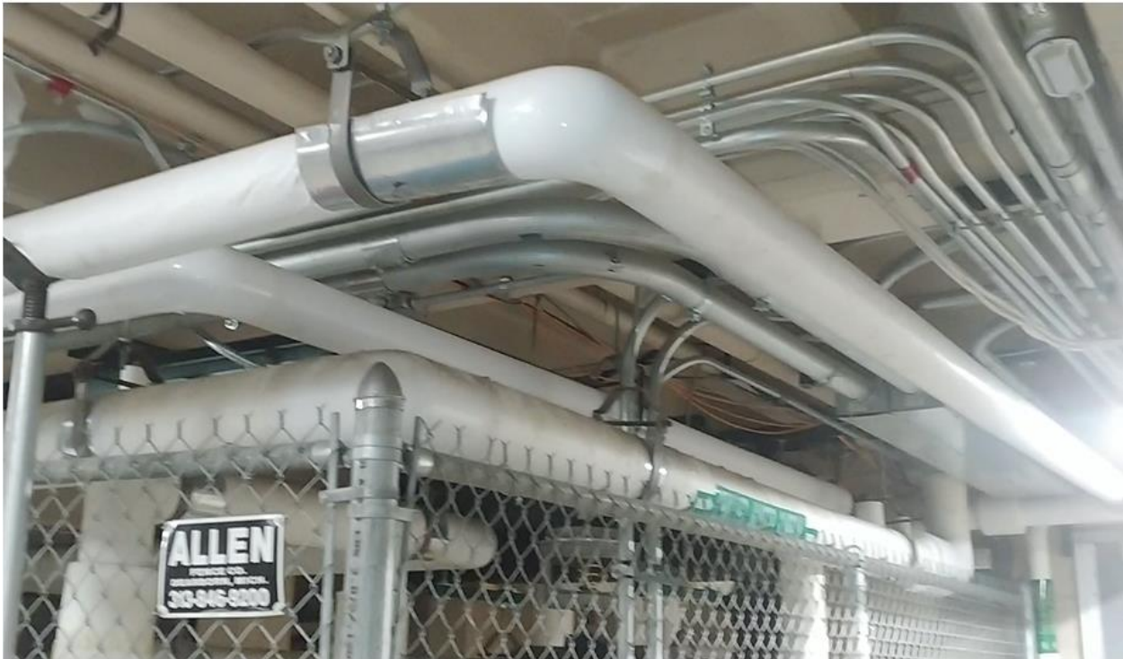
New piping and old piping future connection location
